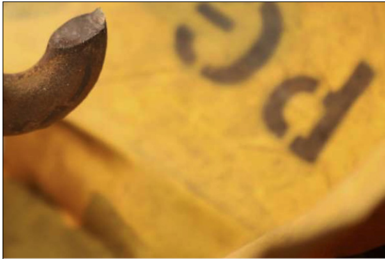
Pacific Gas and Electric Co. has released a photograph of the broken hook on its Butte County power tower involved in the ignition of the deadliest and most destructive wildfire in California history in 2018 (Source: U.S. District Court).
