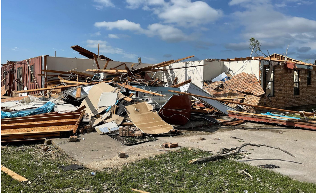
A house that was heavily damaged by the EF2 tornado near Blum, Texas (Source: NWS Fort Worth , May 4, 2021).
