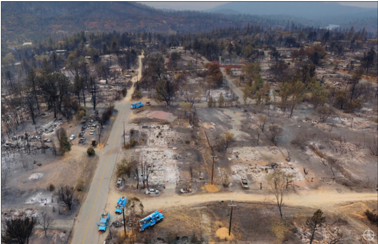
Fig. 1. Santa Rosa CA Wildfire. This is a HANGAR hi-res snapshot, which on a computer can be manipulated in a 360-degree view and zoomed into specific areas. This also reinforces the devastation and total destruction of almost all ground features which makes it difficult to know what area this involves. Agencies are now combining visual imagery with GIS so the drone imagery can be overlaid on geographic layers such as street centerlines and/or satellite map data to provide geographic location identifiers. Source: Courtesy of Alameda County CA Sheriffs Office (2020).
