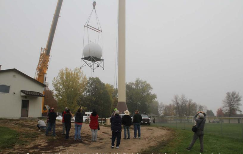
Installation of a new X-band radar in Wendell, MN, which will help fill one of several gaps between weather radars in Minnesota (*Source*: Tara Goode, October 19, 2023).
